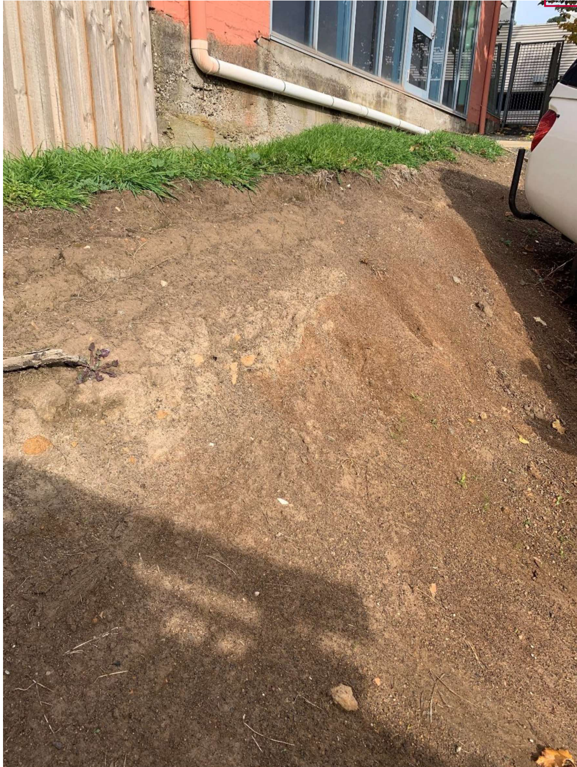
Figure 10: Cutting in front of former workshop
