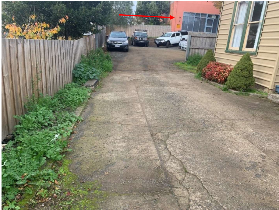
Figure 9: Driveway of 63 Frederick St showing old workshop (pink) and location of cutting
