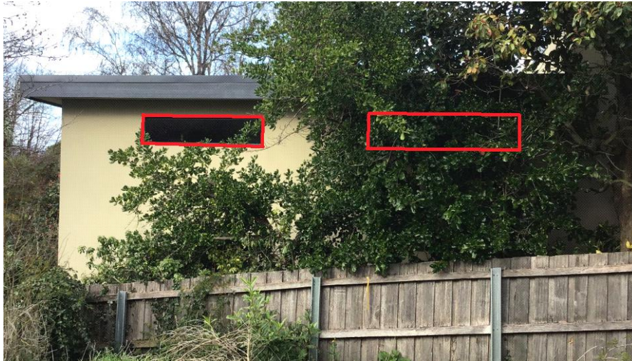
Image 2 - Recreation room windows in red
