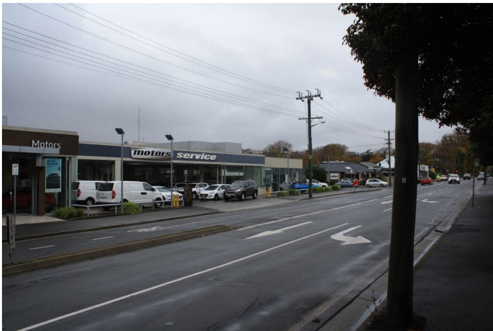
Figure 21 - Motors Services on the North-Eastern Side of Margaret Street Adjoining Hyundai Motors, Taken From the South-Western Side of Margaret Street (taken 10/05/2021, 1.8m above ground. Canon EOS100D. ISO 800. 1/125 Sec. f/7.1 18mm)
