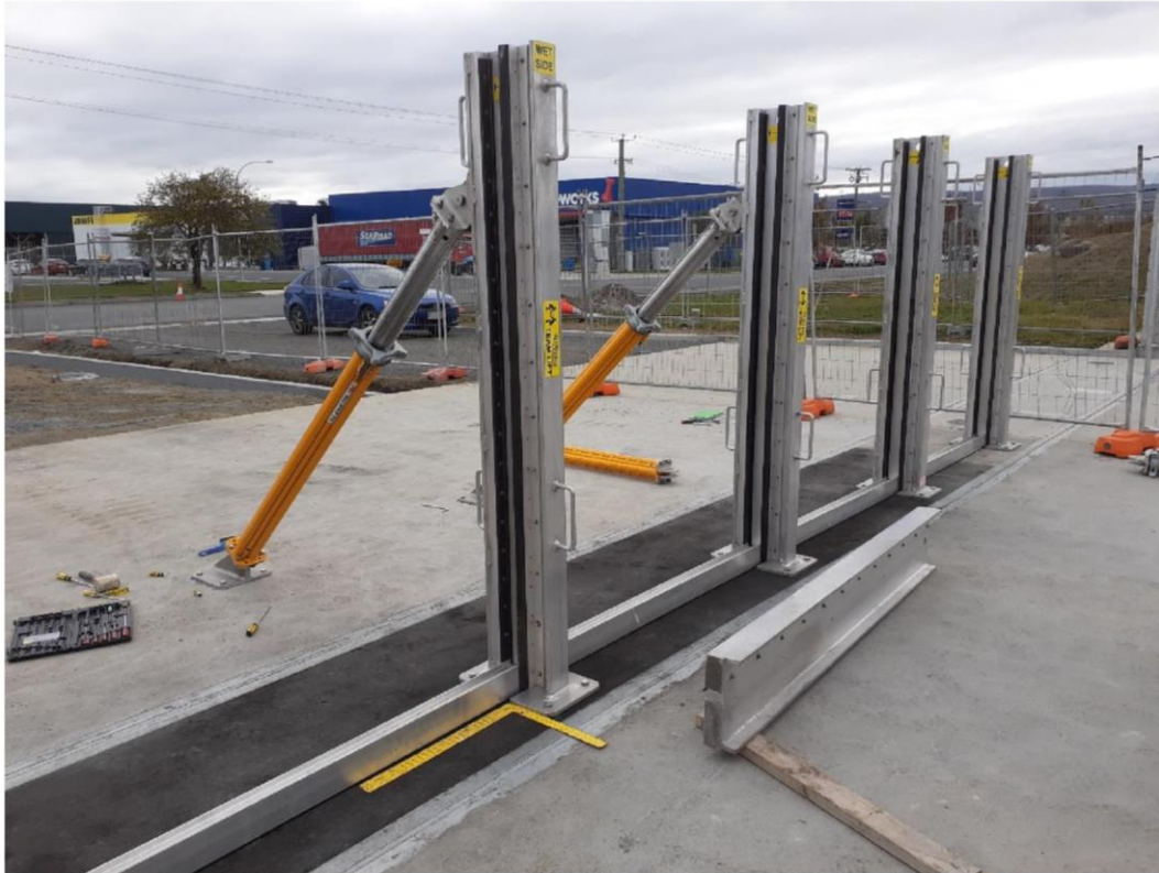
Kings Wharf Levee (Taroona St.) Floodgate - construction is close to completion
