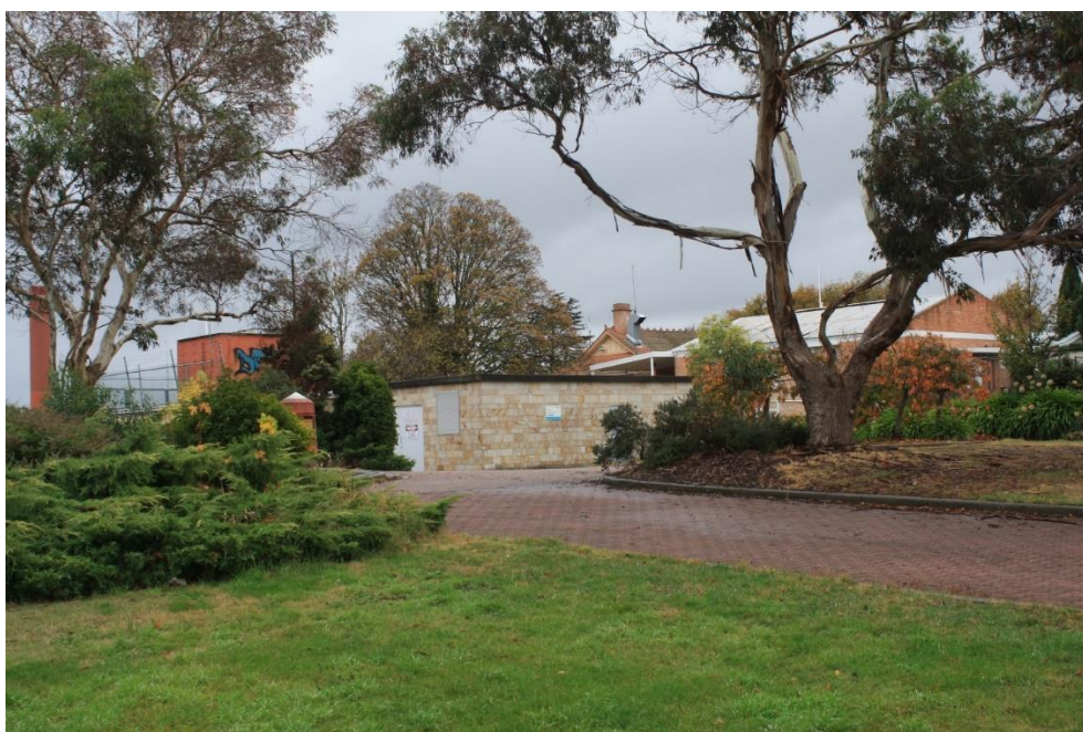
Figure 13 - Pump Station in Kings Park Taken From the Northern Side of Paterson Street Facing North (taken 10/05/2021, 1.8m above ground. Canon EOS100D. ISO 800. 1/125 Sec. f/7.1 18mm)
