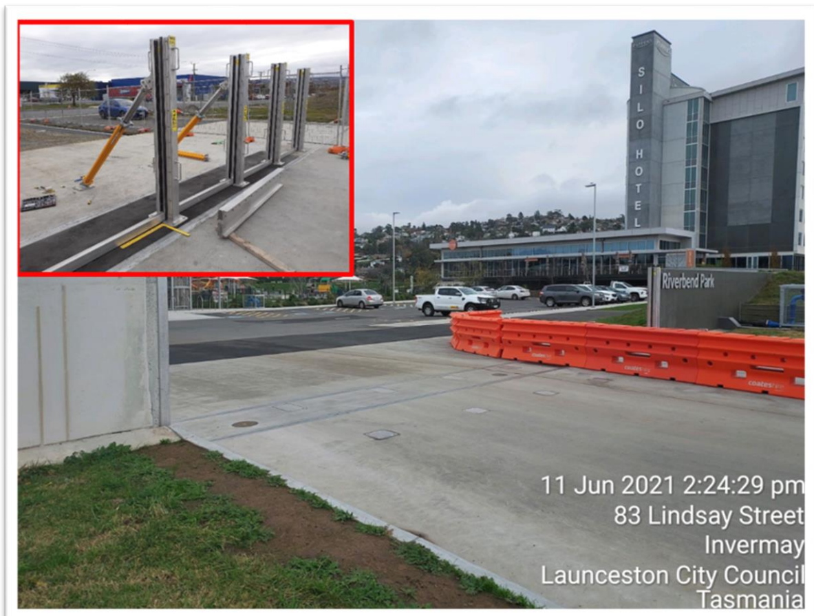
Kings Wharf Levee: New Bauer gate at Riverbend Park entrance
