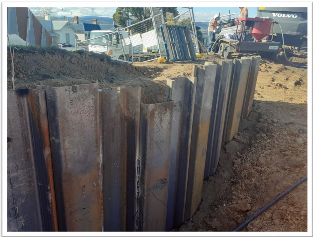
Steel piling installation upstream of Charles Street Bridge, August 2021.
