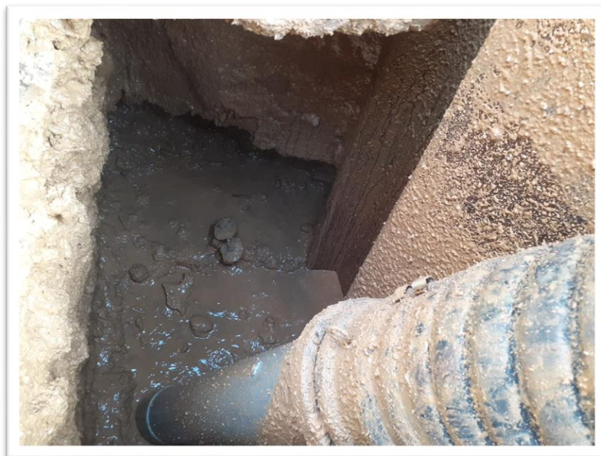
Bentonite plugging upstream of Charles Street Bridge, August 2021
