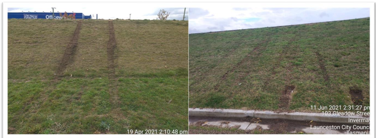
Four-wheel drive vehicle causing damage to earth levees during winter 2021
