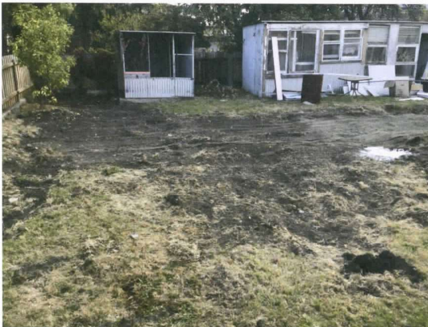
Depth of topsoil removal more is more readily seen in this image particularly in front of the existing aviaries and near the base of the lemon tree at left near the rear boundary.
