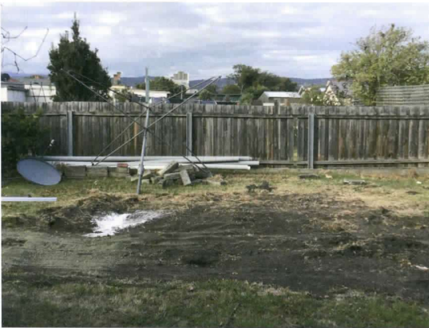
Excavation images of the backyard of 23 Lytton Street showing the removal of topsoil prior to refilling with blue metal.
