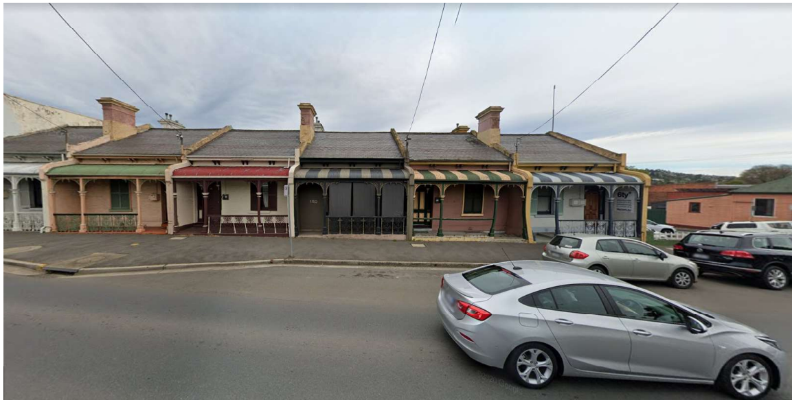
Figure 2.2: 152 Bathurst Street is the dark grey central terrace unit. (source Google Street View: image capture Oct 2019)
