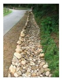
See photo of existing open drain on eastern side of driveway. Water to run from left to right of image into proposed rock drain.
