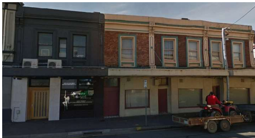
7-11 Tamar Street – GPA Photo 2018
