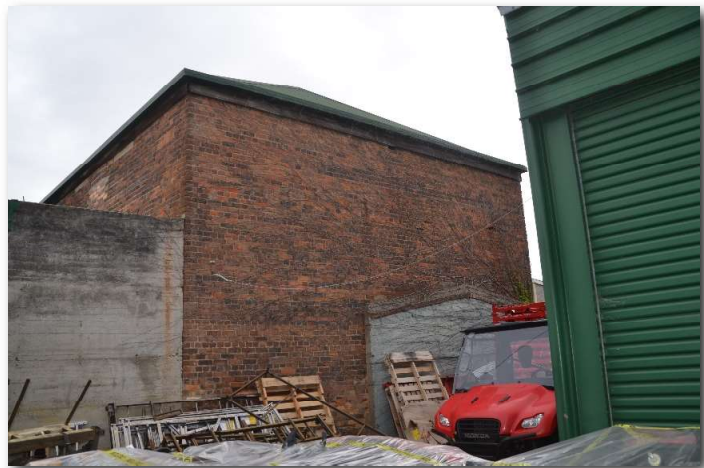
Rear of building directly behind Boland St Site - GPA Photo 22-3-2018
