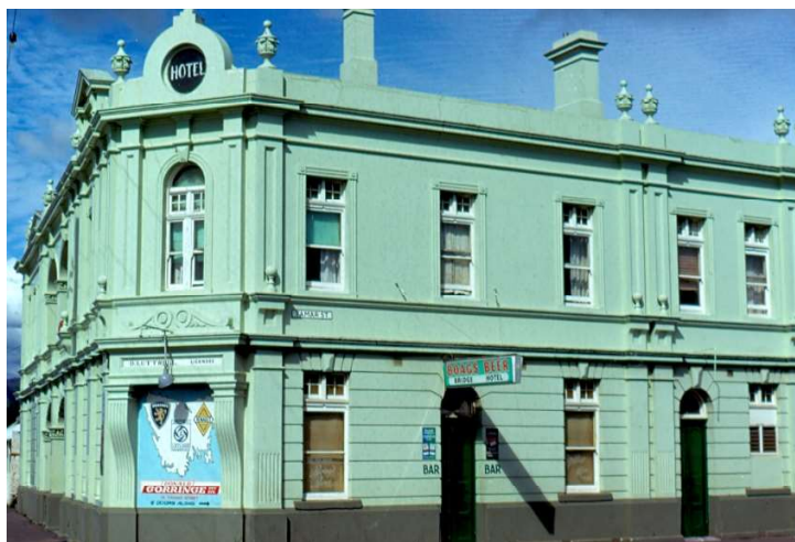
1940s as Victoria Bridge Hotel - Libraries Tasmania LPIC 33-4-119
