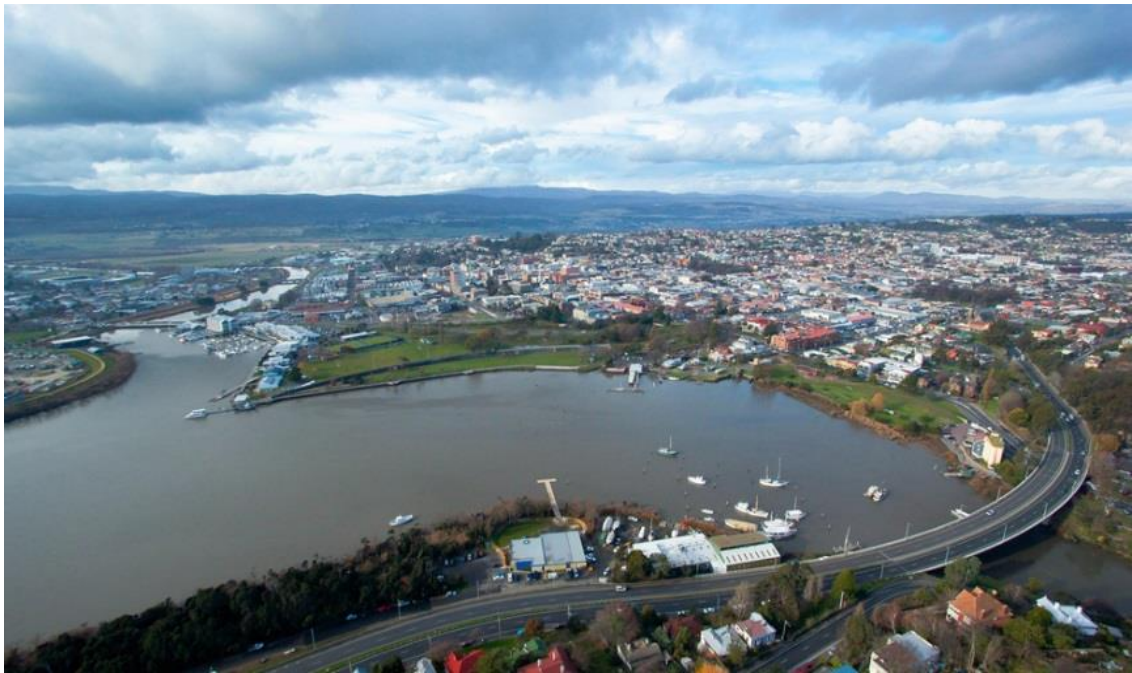
Figure 3 View of central Launceston from north-west
