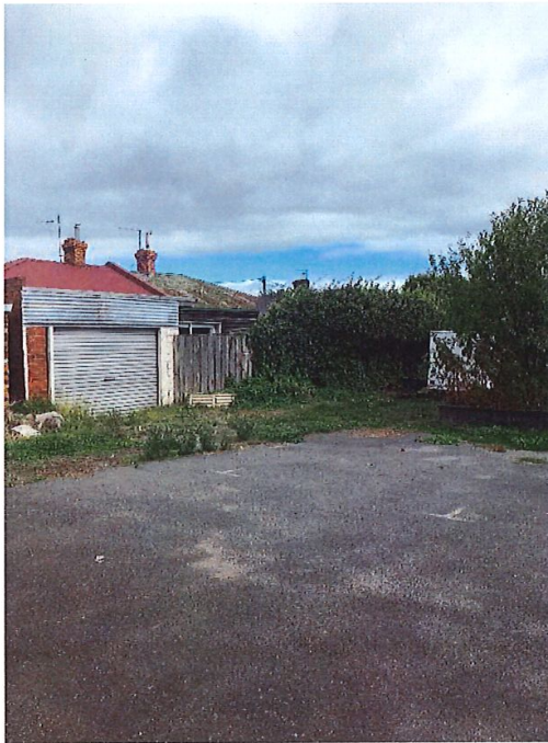
REAR OF 24, 26 BEDFORD STREET – NORTH FACADE
