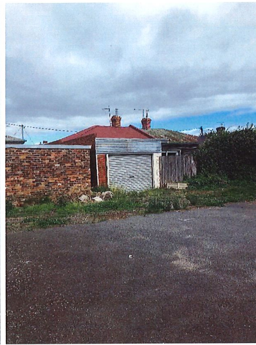
REAR OF 24 BEDFORD STREET GARAGE (BRICK BOUNDARY WALL TO SHED ON 22)
