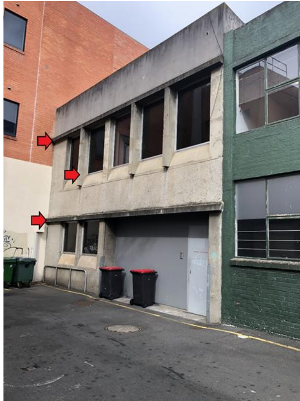
Figure 2. Historical photograph (indicating the protrusions in red)
