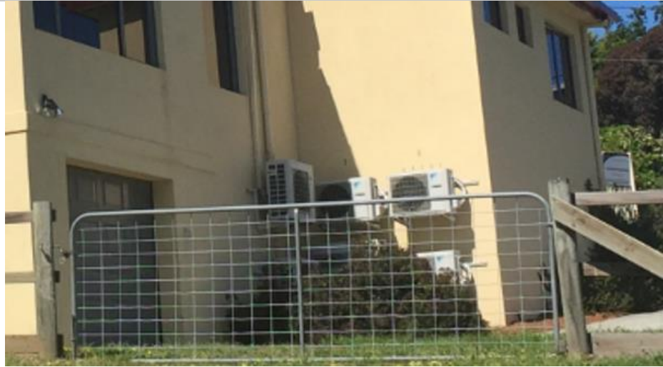
Condenser units on the existing dwelling located 5.5m - 7m from proposed internal road.
