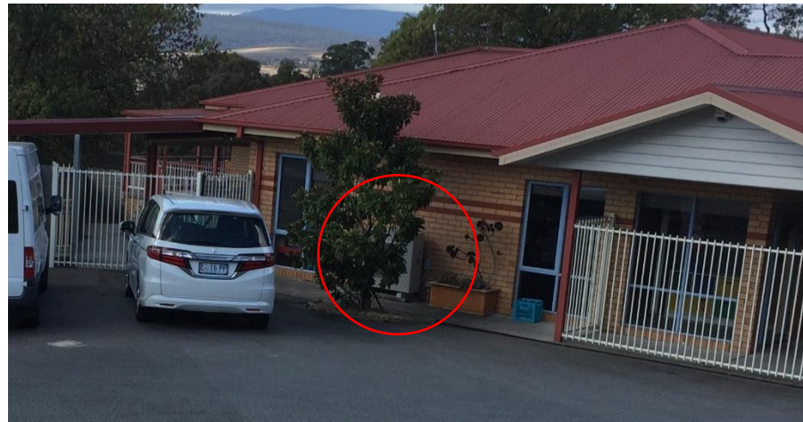
Condenser unit for the respite centre located behind tree. Separated from respite centre 2 by approximately 8 metres.
