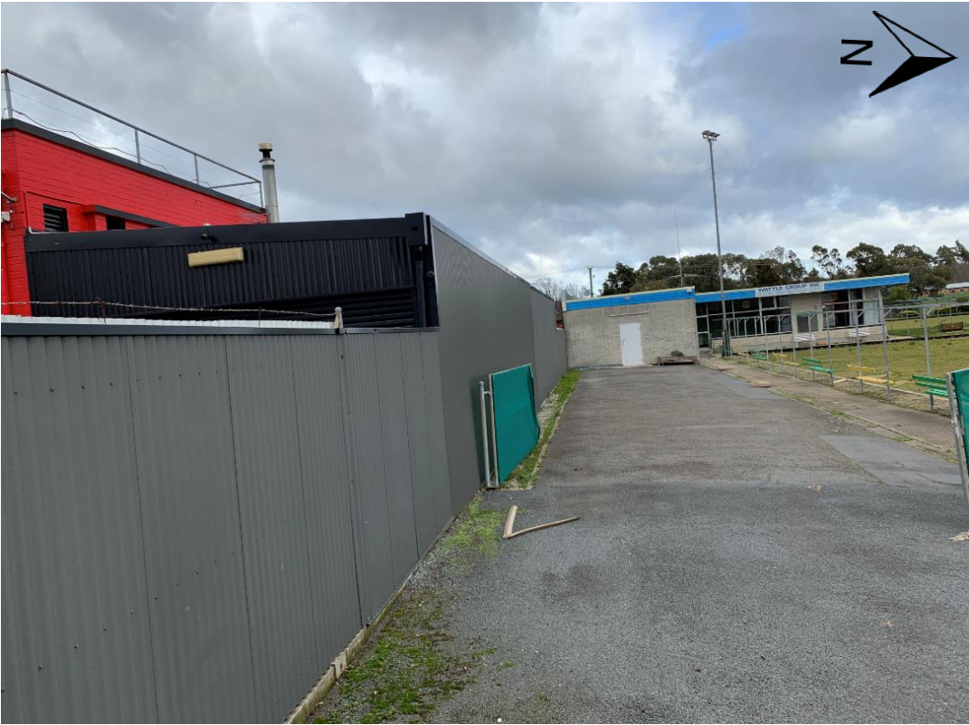
Figure 15: Driveway, former clubrooms and adjacent tattoo studio
