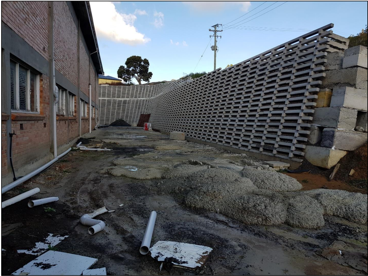
Figure 19: Retaining wall at Lot 1 and Lot 2
