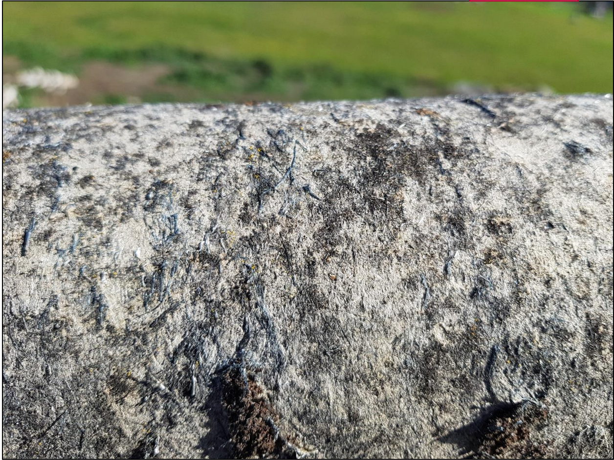
Figure 15: Asbestos Super Six Roof Ridge Cap at 45-47 Thistle Street West – Loose Asbestos Fibres
