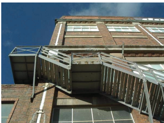
Part of the Glen Dhu Street elevation: steel fire stair, face brickwork with concrete lintels, steel framed windows, and recessed downpipes
