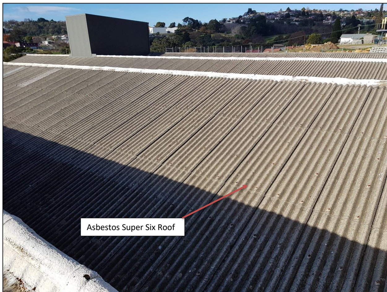
Figure 14: Asbestos Super Six Roof – 45-47 Thistle Street West
