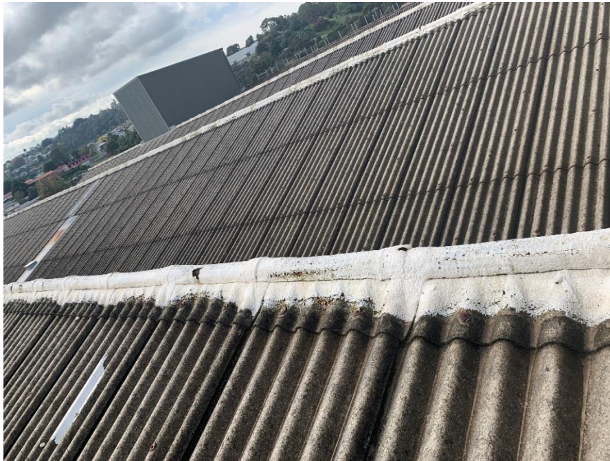
Figure 1 Super 6 Roof indicating maintenance
