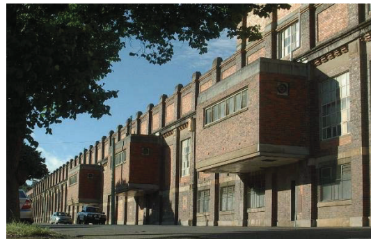
Projecting ablutions blocks on Glen Dhu Street
