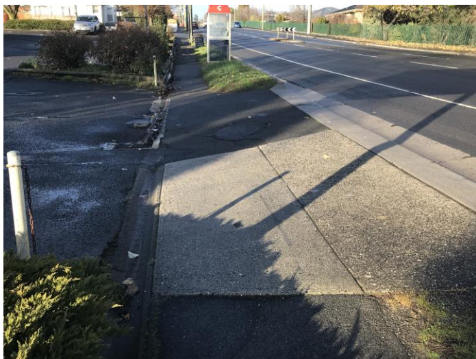
Figure 8 Looking south across #359 access
