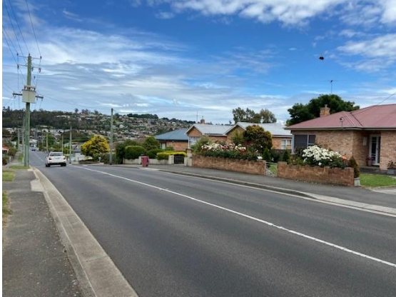
Figure 13 Frontage to Opossum Road for adjoining properties to subject site
