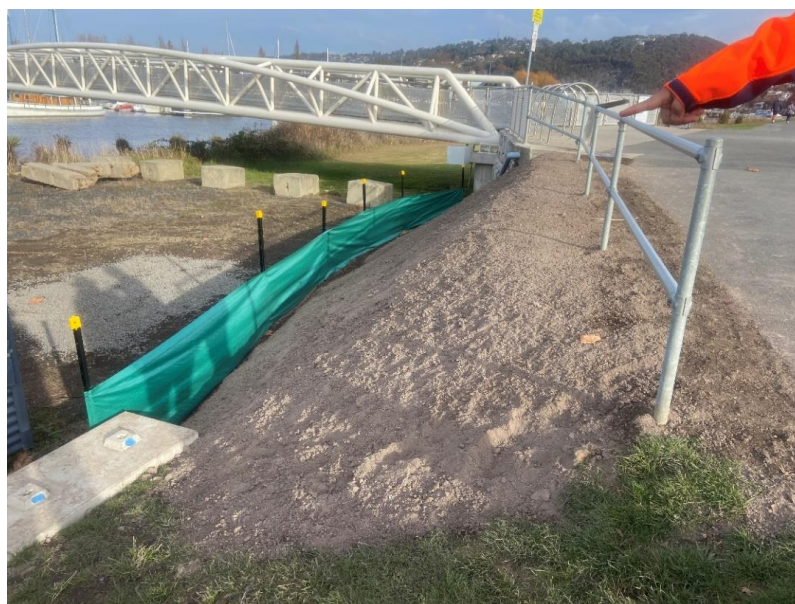
Site of Riverbend levee erosion after intervention
