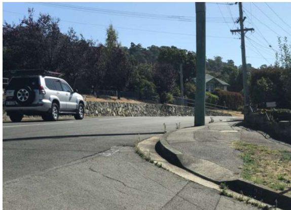
Figure 18 – Looking right along Connaught Crescent from Connaught Place.
