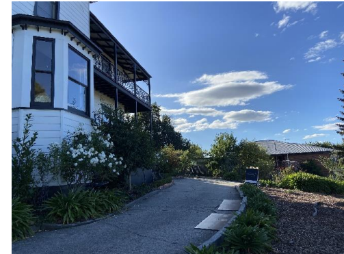
Figure 5 Existing 2 storey building and access for visitor parking
