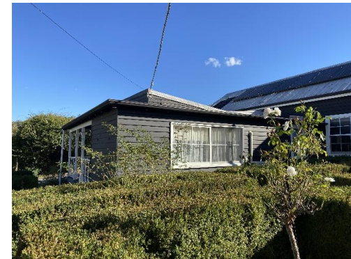
Figure 8 Existing rear building showing section to be removed
