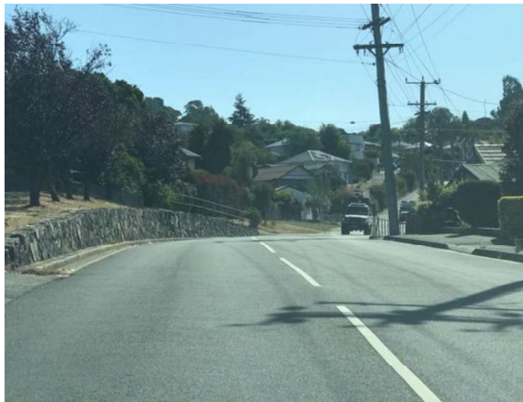
Figure 21 – Connaught Crescent Eastern approach at Connaught Place.
