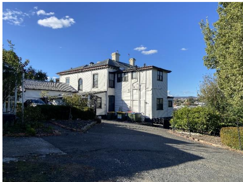
Figure 6 Existing two storey building from rear of lot
