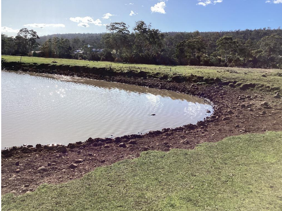
Figure A3-2: Existing dam toward the centre of the title.
