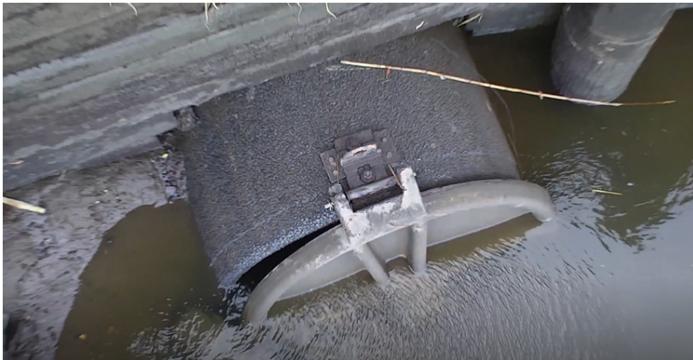
A broken tide flap identified with drone surveillance
