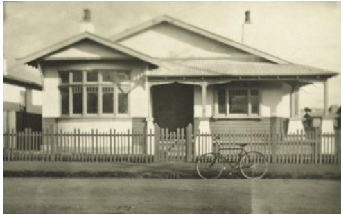
Figure 11 - View of 15 Mayne Street (Libraries Tasmania NS3484-1-78)
