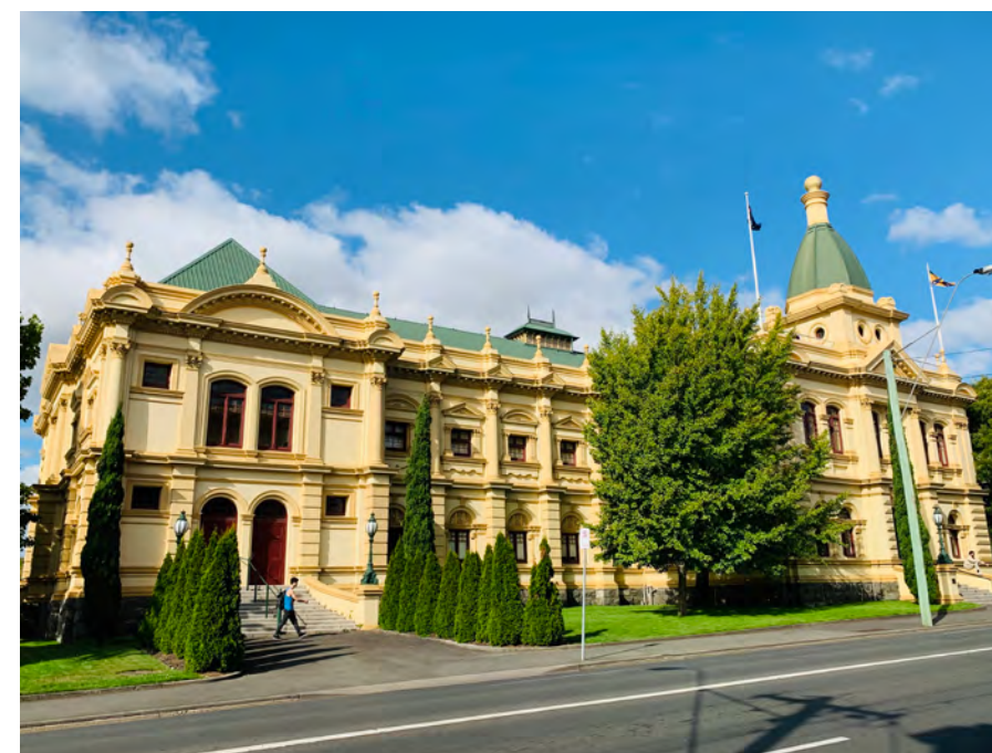
Tamar Street elevation (north end).
