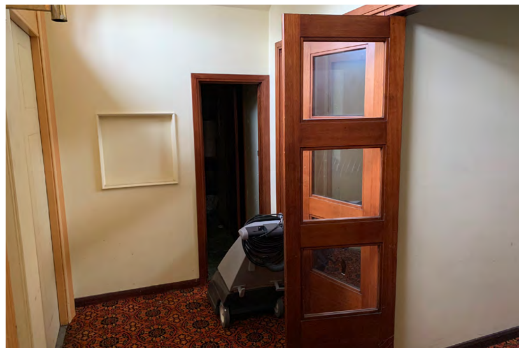
Toward Cleaner's Store from Lobby.
