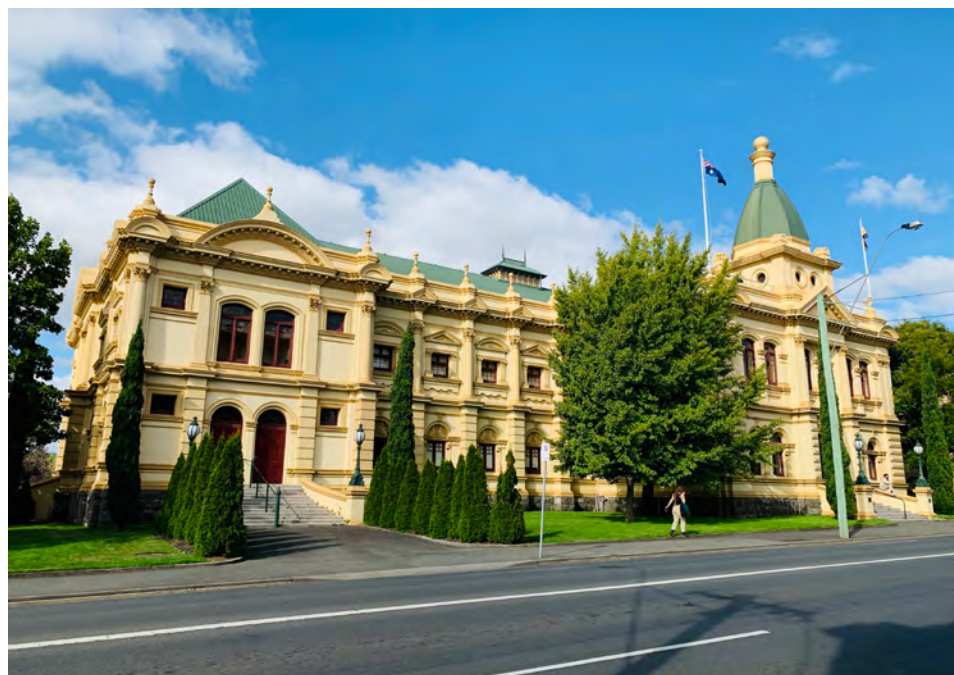
View E: View south east from across Tamar Street level with the North Wing
