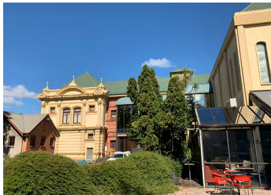
The south end of the rear elevation, with the transition from stucco to brick – the 1980 extension (right).
