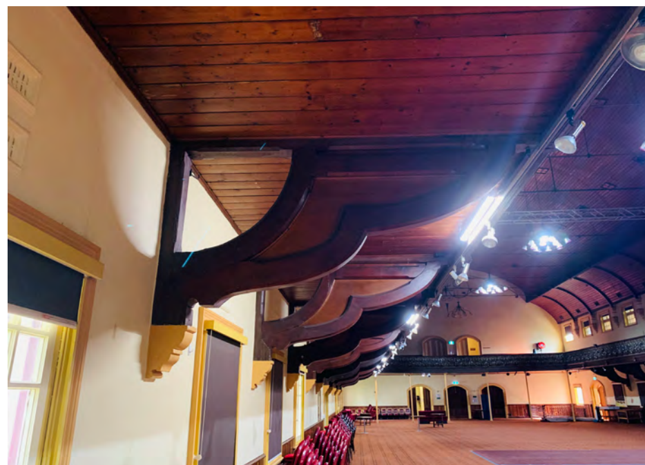
Ground Level view towards the north end detail of Gallery brackets.
