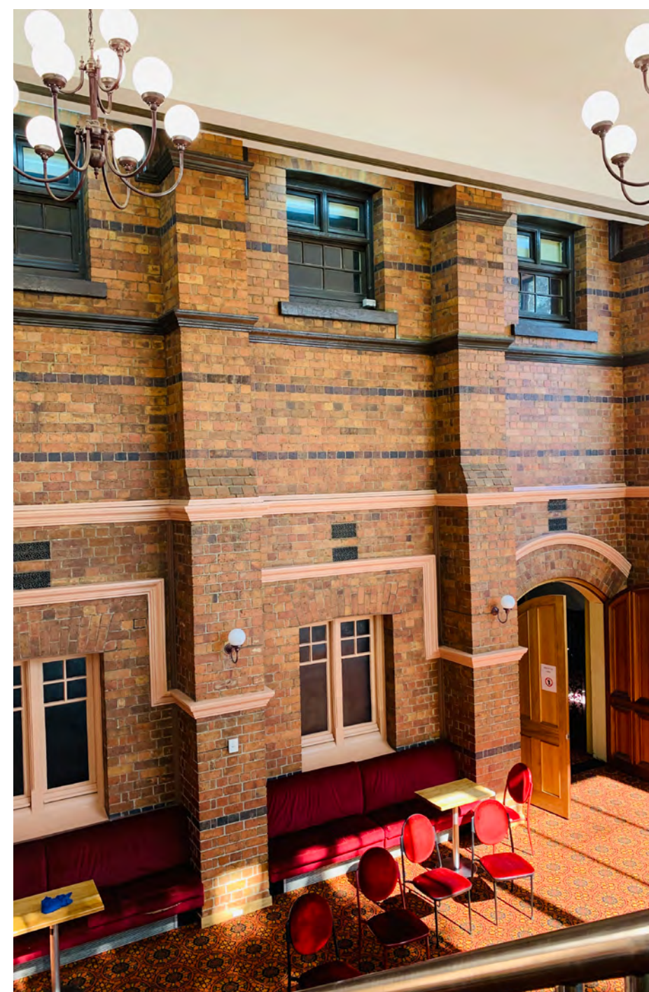
Originally an exterior wall (the rear elevation), this wall is now inside the 1980 extension.
