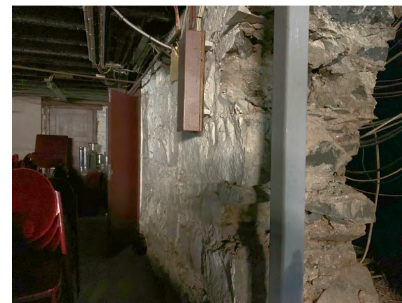
Basement Level store
