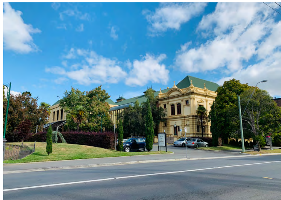
View I: Rear elevation view from Cimitiere Street.
