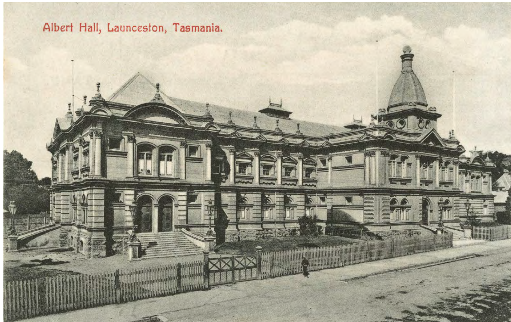
Albert Hall before installation of electricity (Source: unknown, undated, TAHO, AUTAS0016125416552)
