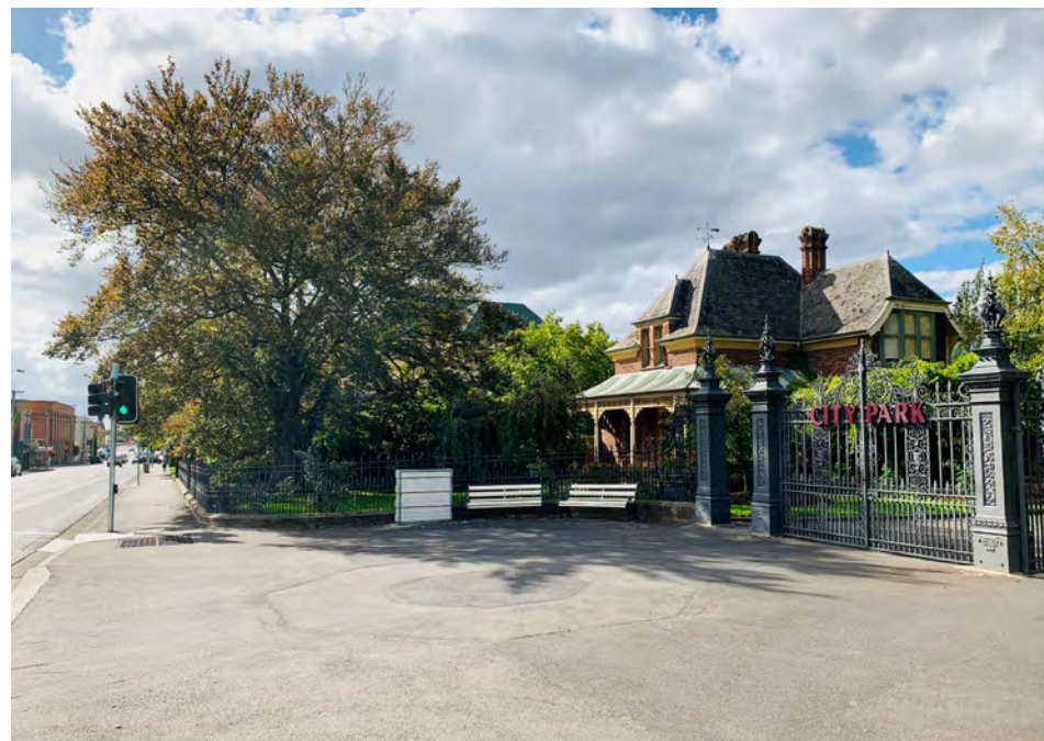
View B: View north from the Tamar St Park Gates, Albert Hall roof is minimally visible behind the trees.
