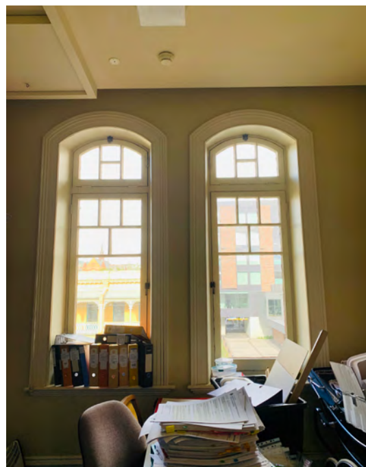
Level 1 Tower Room, view to Tamar Street
