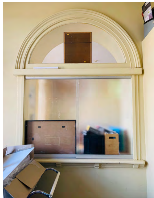
Level 1 Tower Room
