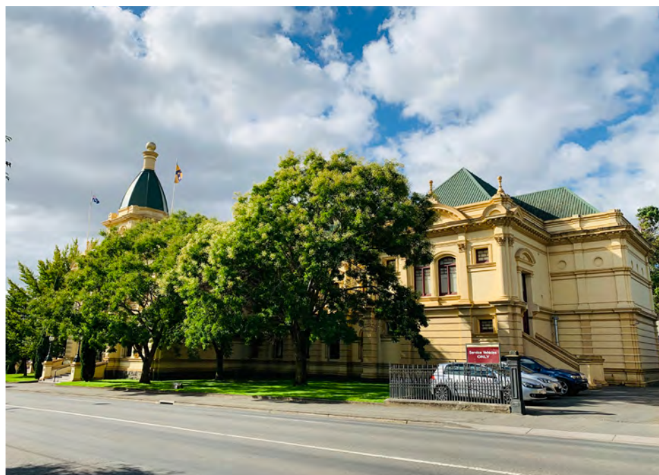
Tamar Street elevation (south end).
