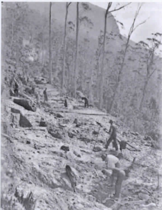
1930s High ground road building – hand built Central Highlands Tasmania Libraries Tas Online Collection NS4023-1-52
