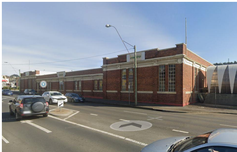
Metro building on Wellington street
