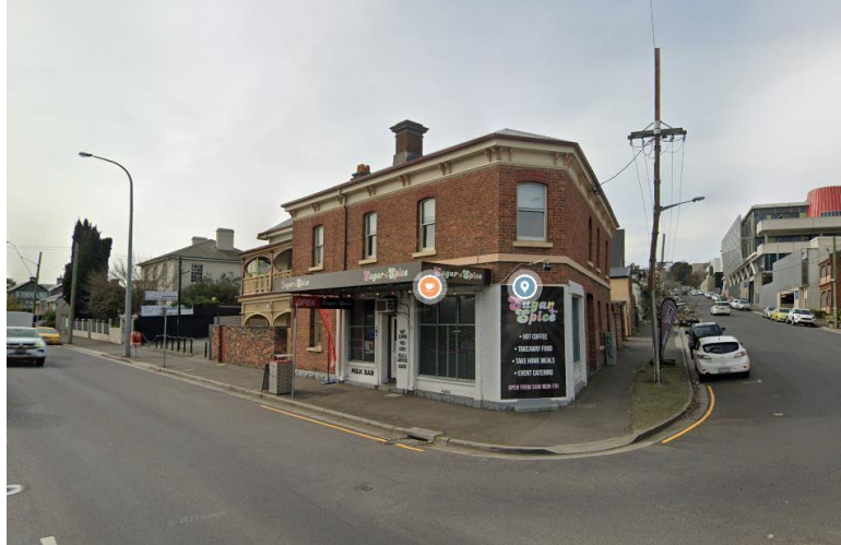
76 Frankland st heritage listed building
