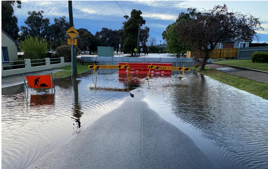
Figure 4 - Hart St Gate (NG1) leaking during October 2022 Flood
