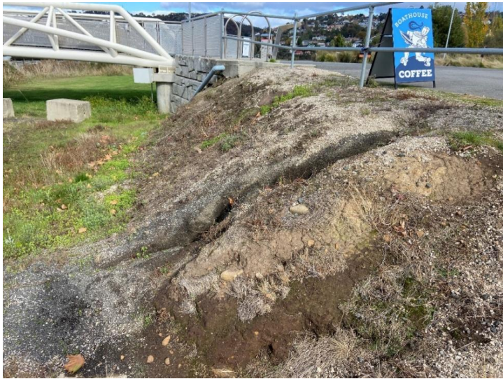
Figure 7 - Site of Riverbend levee erosion before intervention
