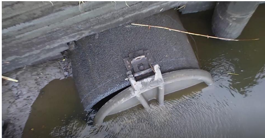
Figure 18 - The broken tide flap identified with drone surveillance
