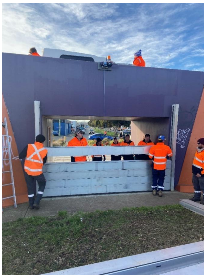
Figure 17 - Closure exercise of Holbrook Street Gate/Telstra gate (IG2), placing one of the logs. August 2024
