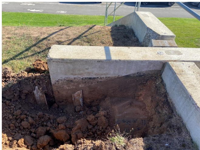
Figure 9 - Buried buttress and sheet piling visible at the junction of the concrete wall and wing wall
