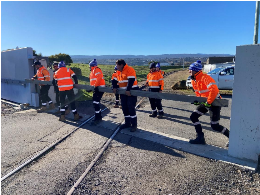
Figure 15 - Closure of the Glebe Farm Gate (EG1). The length and weight of this log is of concern and is planned for rectification. August 2024
