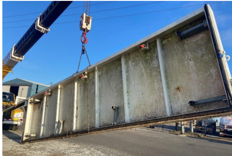
Figure 2 - Gate being craned off prior to upgrade
