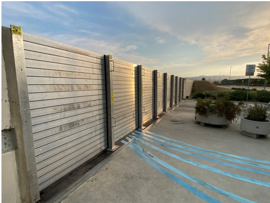
Installed flood gate, viewed from the wet side
