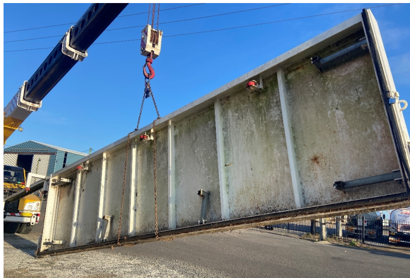
Gate being craned off prior to upgrade
